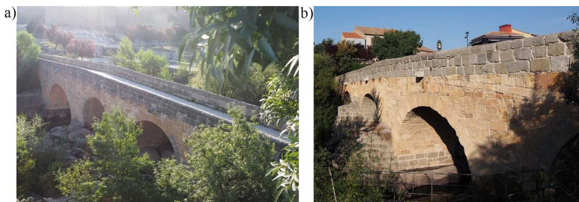
171 Figure 1. General view of the bridge: a) upstream and; b) downstream. 172
